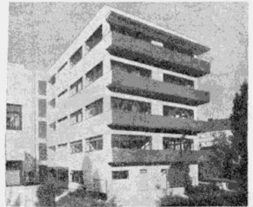
Brno studentu nams. Architekts Bohuslavs Fukss.
