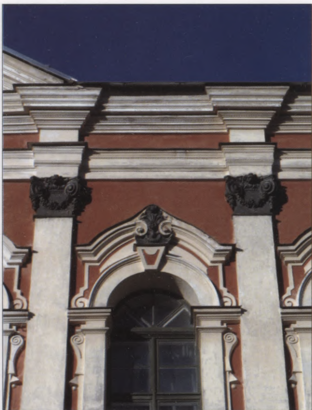
108. Dienvidu fasādes fragments Fragment of the southern façade
