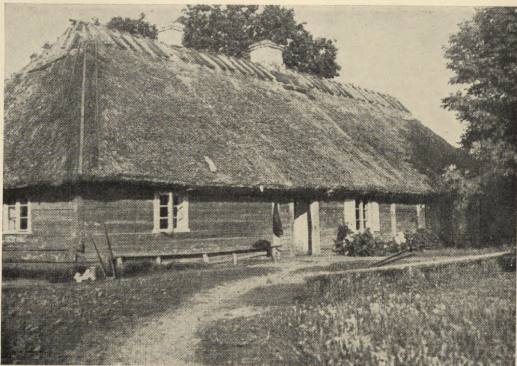
An old farm house in Kurzeme. Early Latvian farm-houses were built of round or square timbers and thatched with straw, reeds or wood bark. The middle of the house was occupied by a section known as the nams , i. e. a room with a hearth. On either side, separated from the nams was a heated living room.
