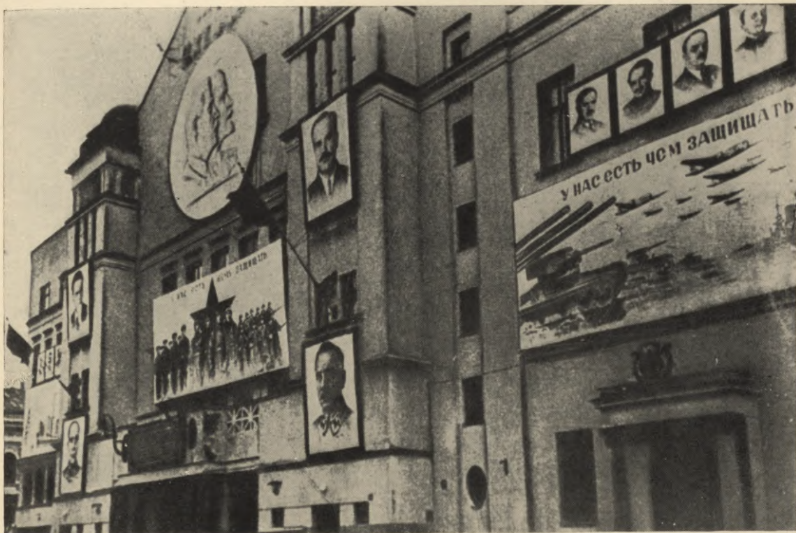
The Year of Terror: the House of the Latvian Society, Rīga, in 1940. For the Russians to cover the face of this house with their bolshevik propoganda in such a manner as may be seen from the illustration above was a deliberate affront to the national pride of the Latvians. The Latvian Society played an important part in the National movement during the latter half of the 19th century and later during the twenty years of independence.
