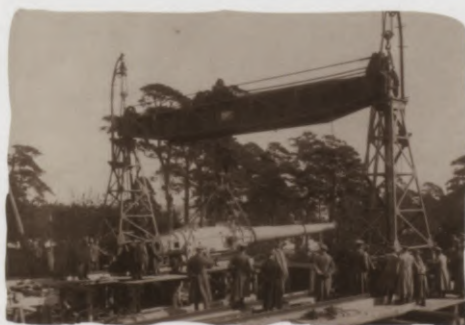
Krasta artilērijas lielgabala demontāža Dismantling of the Coastal artillery cannon
