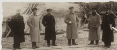
Inženierkapteinis Aleksejs Židkovs (1859.-1932.) ar celtniekiem Captain-Engineer Aleksey Zhidkov (1859.-1932.) and constructors
