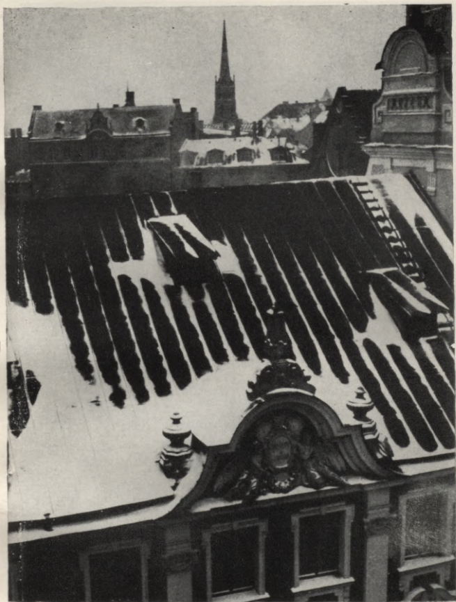
Roof of the old church, looking from the street.
