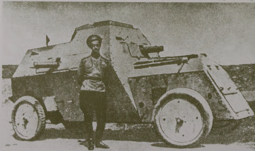
An armored car of the Russian Army. Manufactured at the Izhora factory in St. Petersburg on a "Russo-Baltique" chassis. 1915.
