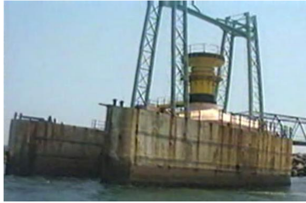
Fig. 3.1. Indian wave power converter (OWC) [37].
