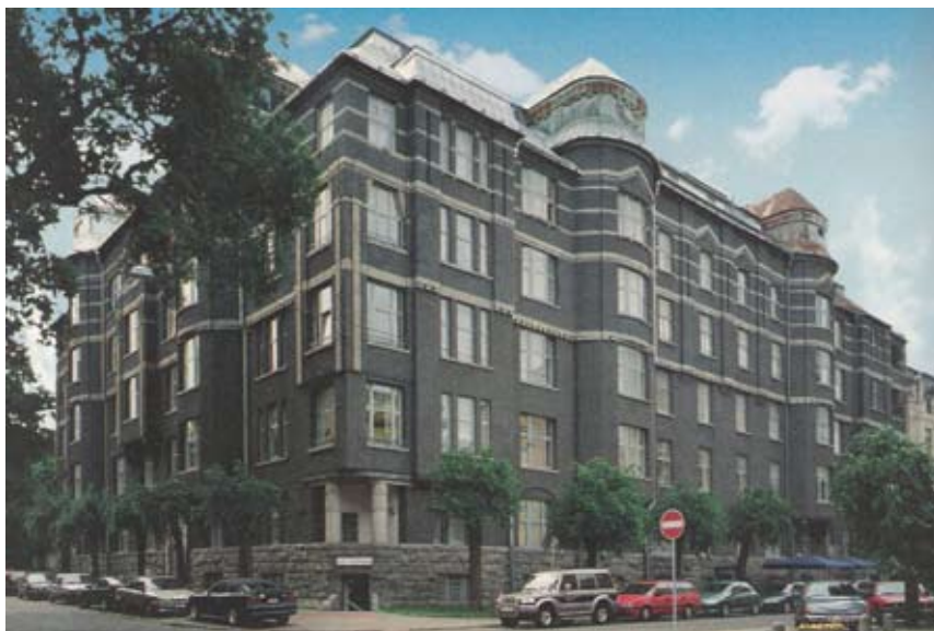
2. Nesterov rental house at 5 Andreja Pumpura Street / 2a Jura Alunāna Street (1906, architects Armas Lindgren, Knut Wasastjerna and Aleksandrs Vanags). Illustration from S. Grosa, Art Nouveau in Riga: Taking A Walk Through Riga in the Art Nouveau Era . Riga: Jumava, 2003, p. 46.
