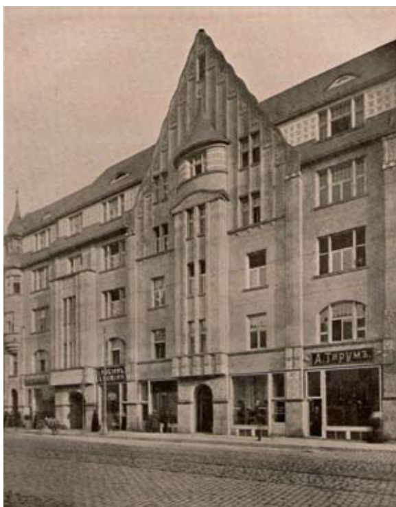
5. Virsis rental and storage building at 62 Brīvības Street (1908, architect Eižens Laube). Illustration from Jahrbuch für bildende Kunst in den Ostseeprovinzen , Riga, 1909, p. 80.
