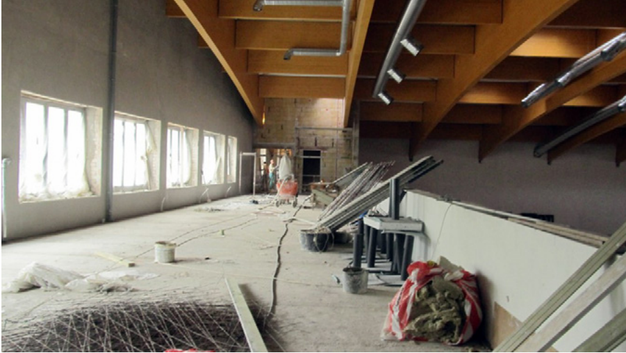
Fig. 7.21. The construction process of sports hall in Palanga city, Lithuania ( www.sporthall.palanga.lt ).
