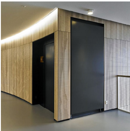
Fig. 3.46. Milling the radiator into wall surface (Hudevad, 2019a).
