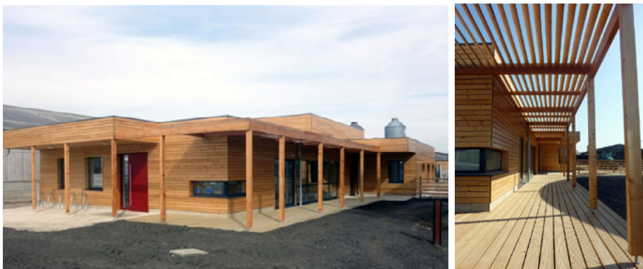
Fig. 1.39. Hadlow College (Passivhaus Trust, 2020).
