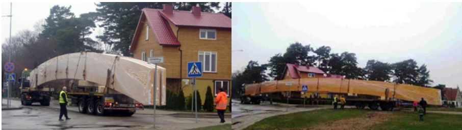
Fig. 7.20. Transportation of 36 m long glulam beams for the multifunctional sports hall in Palanga city, Lithuania ( www.veidas.lt ).
