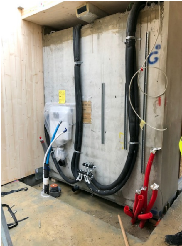
Fig. 3.54. Finished bathroom made of concrete (Byggeskadefonden, 2020).
