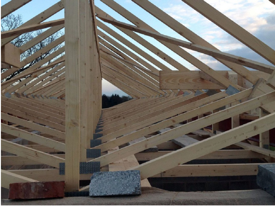
Fig. 6.39. Bracing of the roof (Minera, n.d.).
