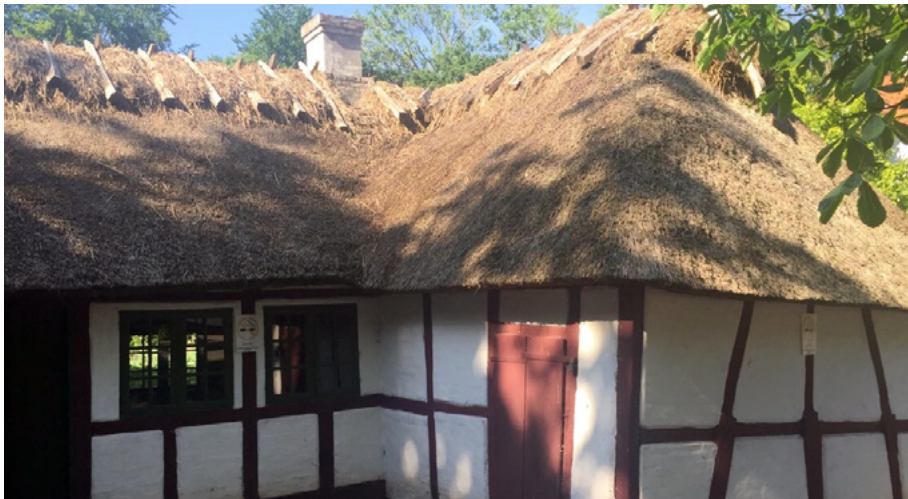
Fig. 3.13. Thatched roof in Denmark, Odense.
