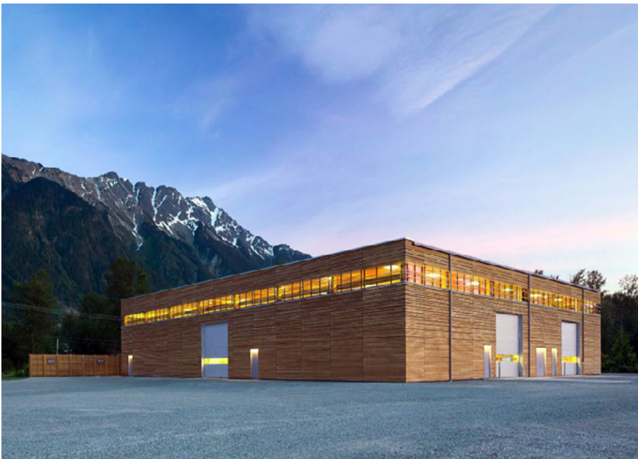
Fig. 1.40. The BC Passive House Factory (McKnight, 2016).
