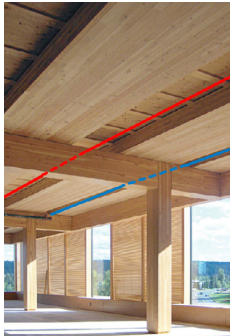
Fig. 3.42. Installations above the beams and between slabs.
