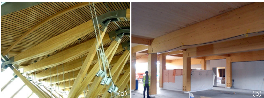
Fig. 2.26. Glued laminated timber, or glulam, is another engineered timber that can adopt varied shapes (a) and achieve very impressive sizes (b): (a) Scottish Parliament, (b) GlaxoSmithKline Carbon Neutral Laboratory for Sustainable Chemistry, University of Nottingham.
