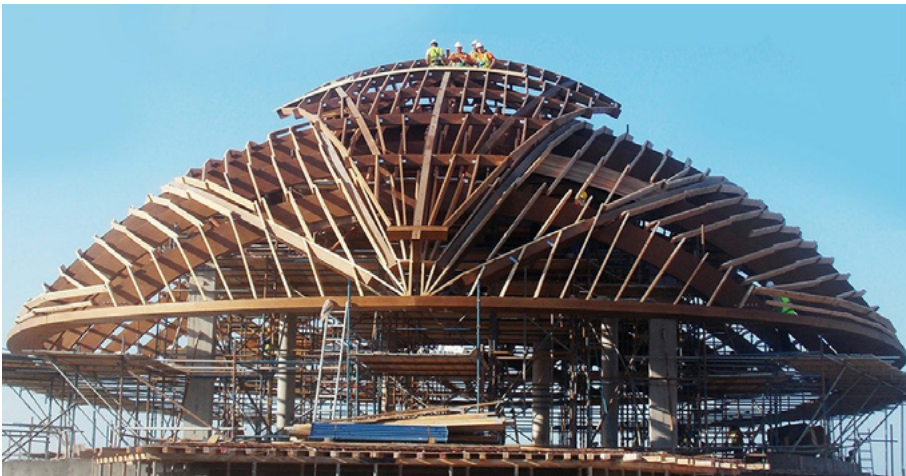
Fig. 7.59. Construction process of the lookout restaurant in Banana Island, Doha, Qatar.
