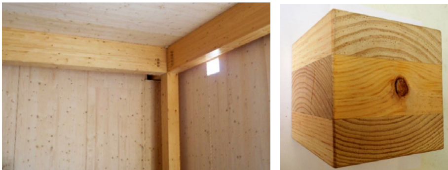
Fig. 2.18. Cross-laminated timber consists of orthogonally glued laminations. It is a versatile product that can be used as a slab or a wall, as seen here.
