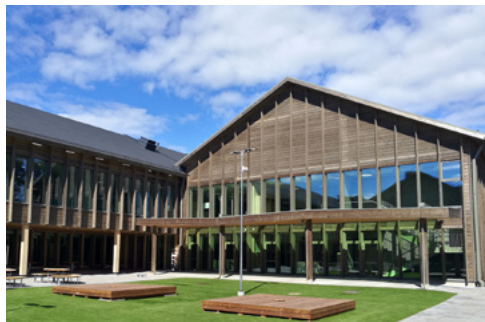
Photograph: Oiva wood Solutions Ltd, 2020
