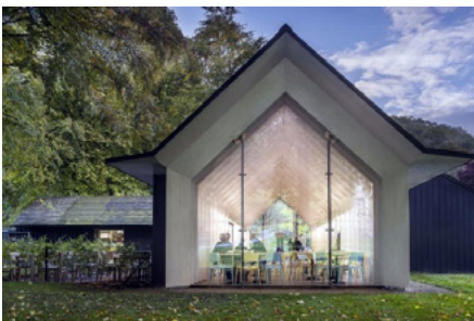
Fig. 7.26. The central hall ( www.e-architect.co.uk ).
