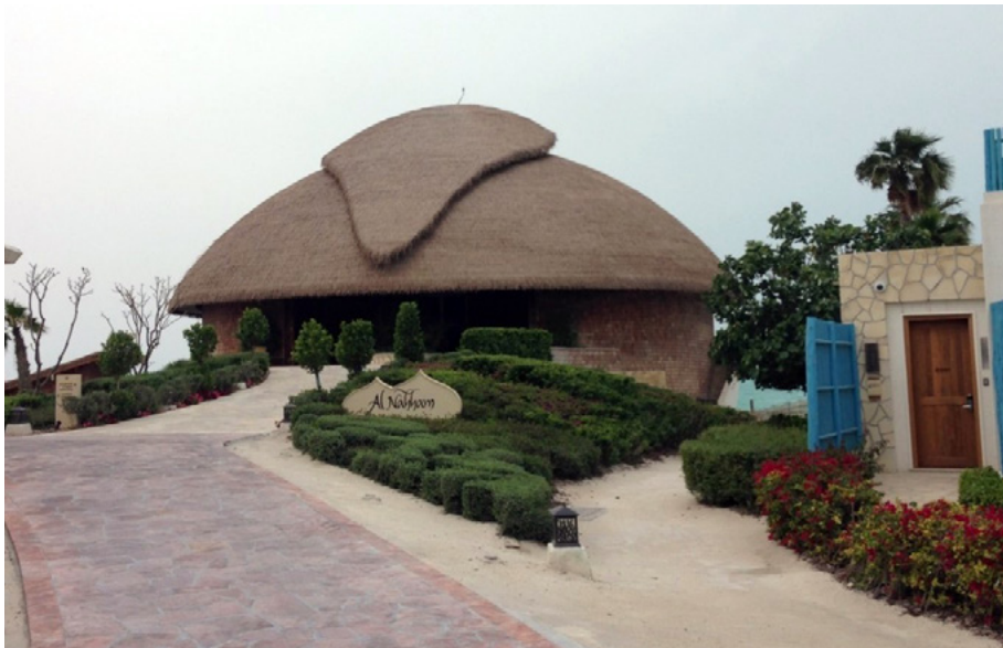
Fig. 7.55. The outside appearance of the lookout restaurant in Banana Island, Doha, Qatar.
