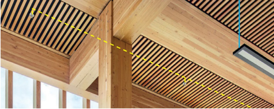
Fig. 3.43. Duct roads closed between the load-bearing CLT slabs.
