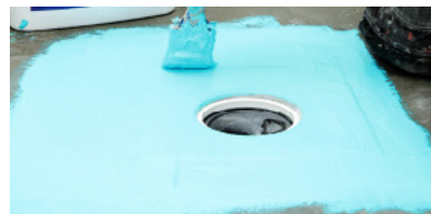
Fig. 3.12. Brushable water proofing in wet room.
