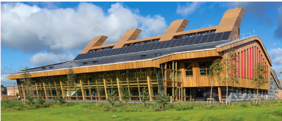
Fig. 1.25. GlaxoSmithKline, UK (BREEAM, 2020).
