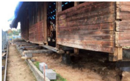
Fig. 7.10. Wooden stands and planking before rebuilding (Gada labākā būve Latvijā 2018, 2019. The best building of the year in Latvia, 2019).
