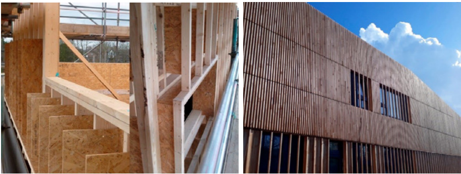
Fig. 1.37. Hackbridge primary school (Passivhaus Trust, 2020).
