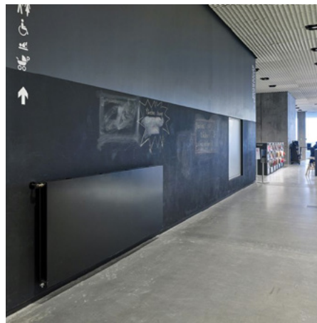
Fig. 3.47. Radiator outside the wall (Hudevad, 2019b).
