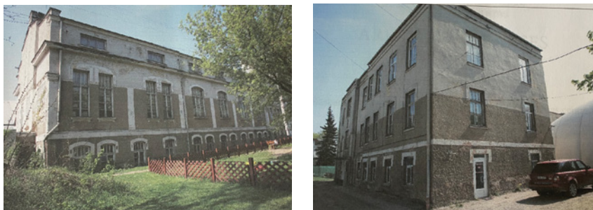
Figure 24. The building at 7 Baldones Street before reconstruction (2009).
