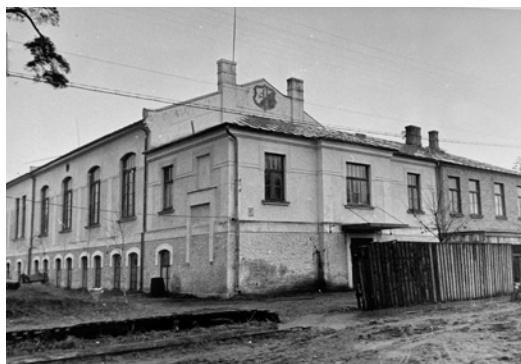
Figure 14. ĀGSS building with a newly built extension (1939).
