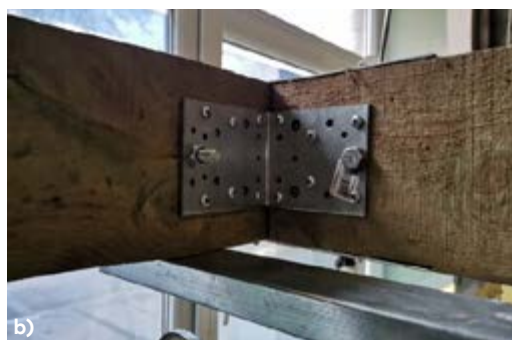
Fig. 1. Timber beams a) and its joint b).
