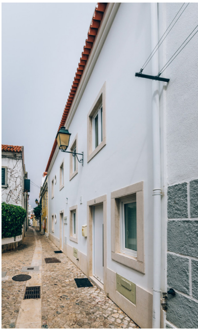
Fig. 18. Rua Santa Vitoria , 4–4 a and 4B, Cascais [Photo: Alexandre Rotenberg].
