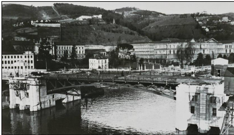
Movable section at an advanced stage of construction.
