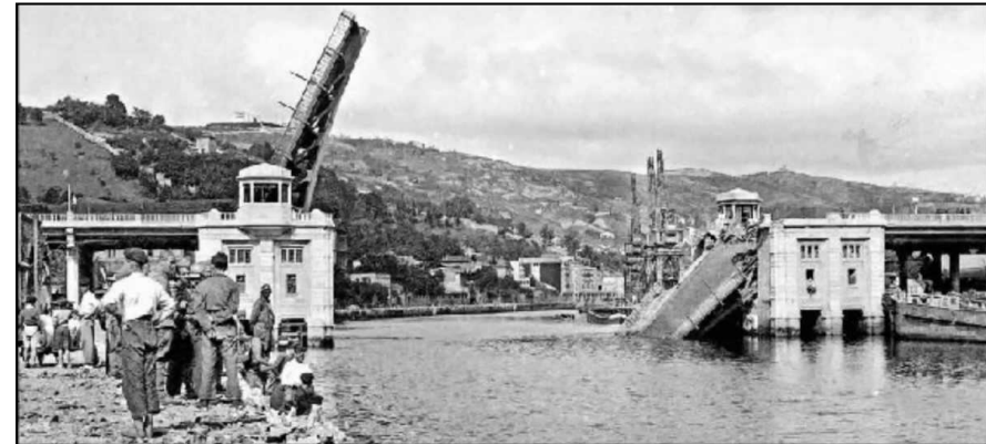
Bridge after its explosion before the imminent arrival of Franco's troops.
