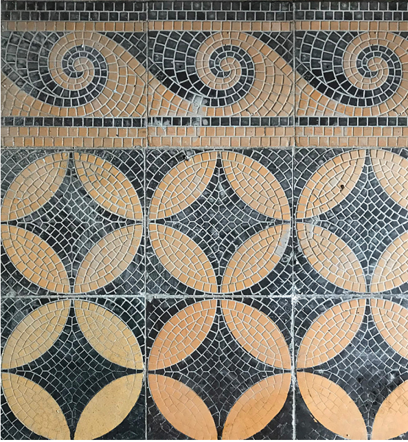
Figure 2. Fragment of floor tiles produced by the Polish company “Marywil” in the vestibule in a building at Rīga, Kalēju Street 14 (arch. Max von Osmidoff). Photo: Agnese Tambaka
