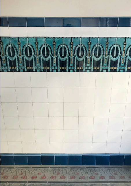
Figure 3. Vestibule at Miķelis Tetere's apartment building at Ģertrūdes Street 60 (arch. Rudolf Dohnberg, 1908). Wall tiles: NSTG, floor tiles: Carl Nevermann & Co Riga. Photo: Agnese Tambaka
